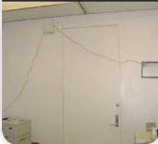
USING EXTENSION CORDS IN PLACE OF PERMANENT WIRING
