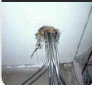
NO FIRE STOPPING IN OPEN PENETRATION
